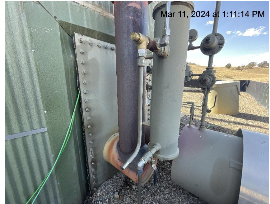
Photo # 9188 PRV vent line on tank burner terminates in an unsafe manner/does not comply with CECMC pressure safety device rules & general safety rules.
