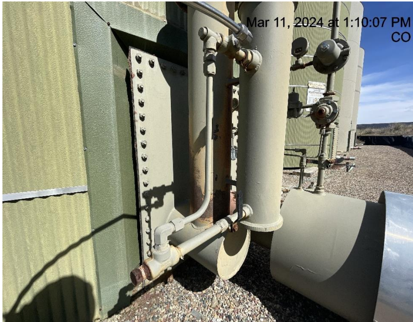
Photo # 9187 PRV vent line on tank burner terminates in an unsafe manner/does not comply with CECMC pressure safety device rules & general safety rules.
