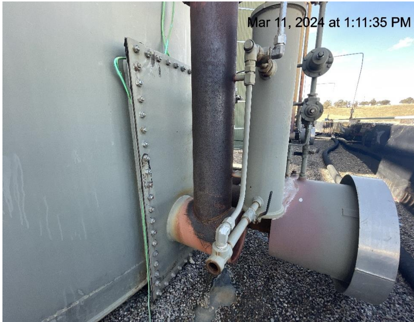
Photo # 9189 PRV vent line on tank burner terminates in an unsafe manner/does not comply with CECMC pressure safety device rules & general safety rules.
