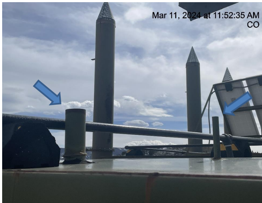
Photo # 9185 PRV vent lines lack caps/do not comply with CECMC pressure safety device rules
