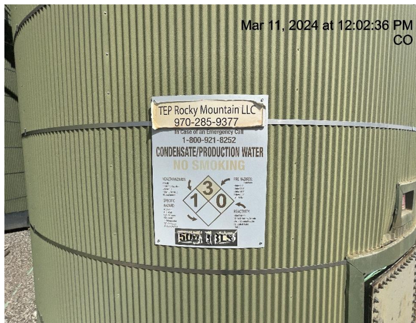
Photo # 9191 Tank label damaged & missing required information
