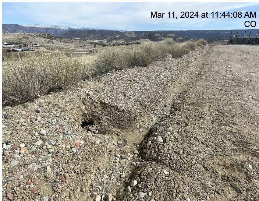
Photo # 9197 Tunnel erosion through berm/BMP needs maintenance
