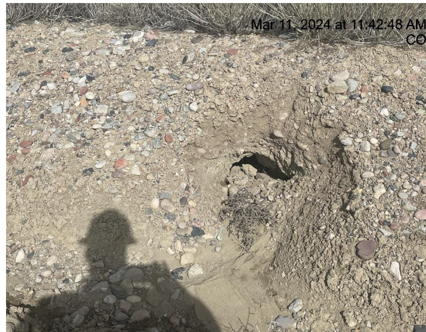
Photo # 9198 Tunnel erosion through berm/BMP needs maintenance
