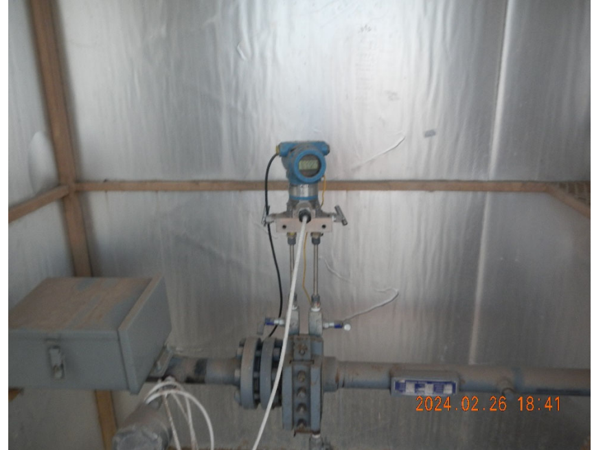
6. Digital gas meter inside meter shed.
