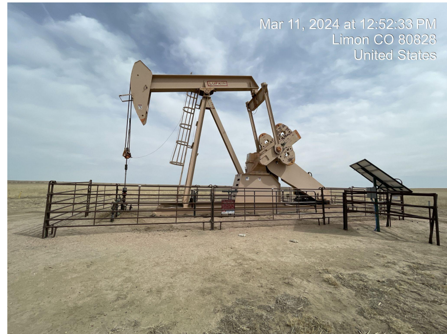
Photo 2. Photo taken facing southeast of wellhead.
