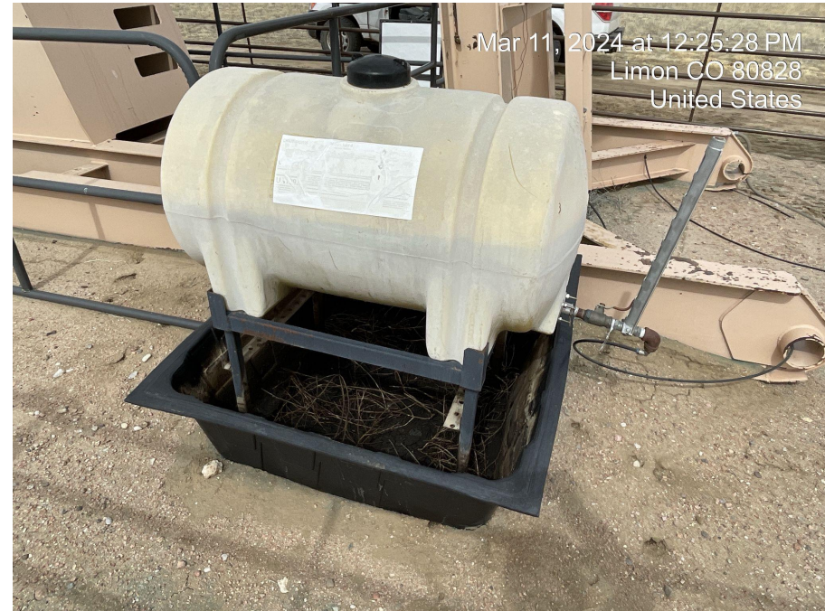
Photo 4. Photo taken facing east of secondary containment without wildlife protection.
