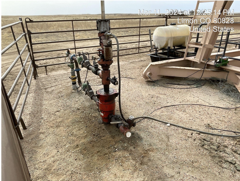
Photo 3. Photo taken facing northwest of staining around wellhead.
