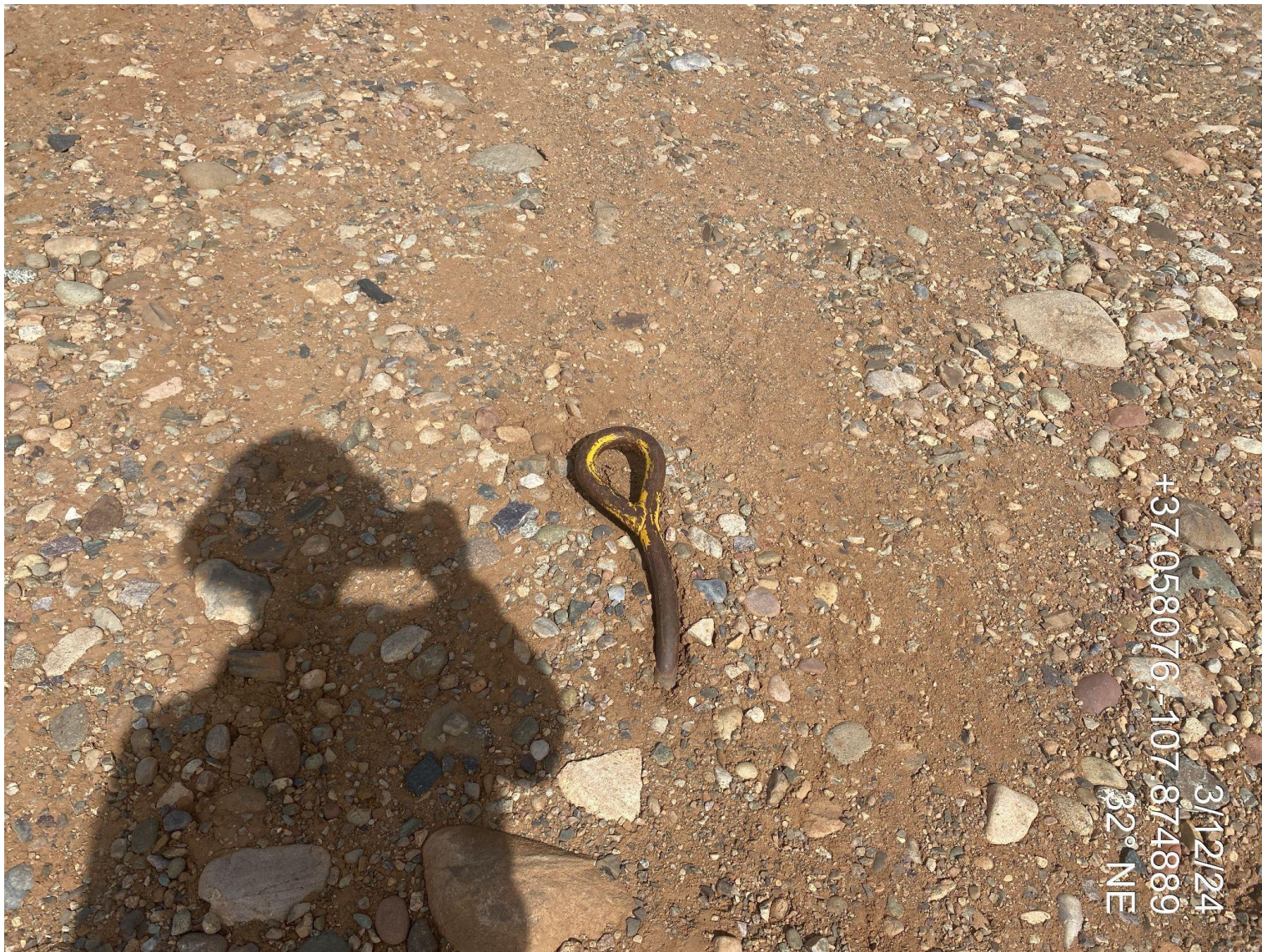
Photo 5. Unmarked anchor guy line observed on location.
