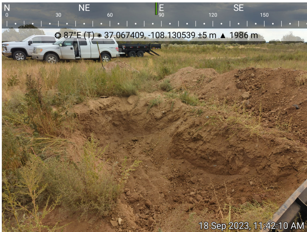
Photo 8: Overall wellhead excavation area, 9/18/2023.
