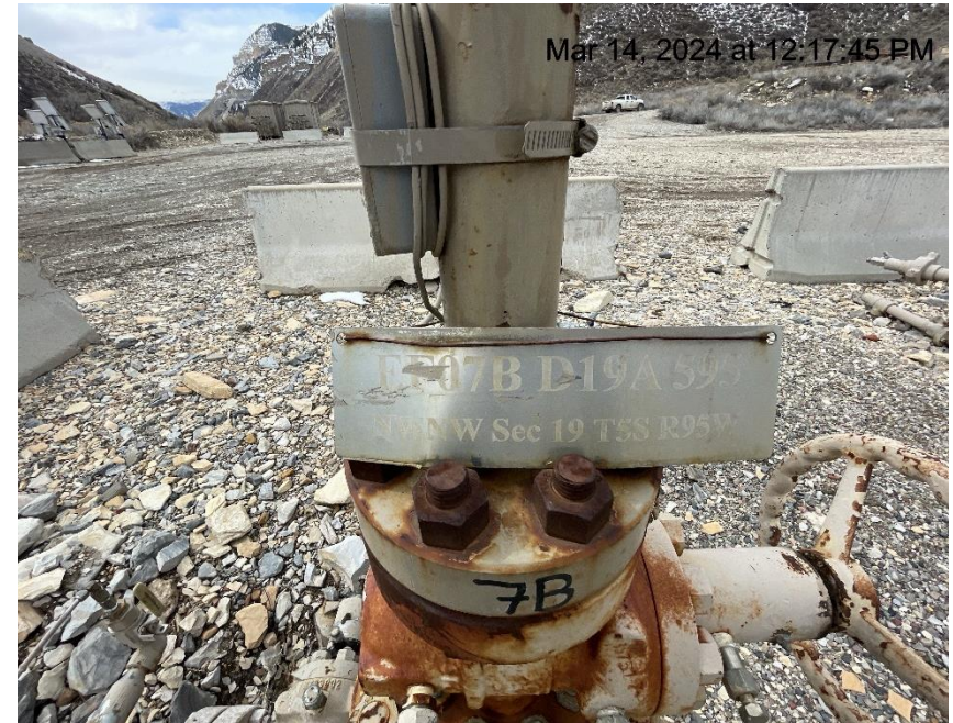
Photo # 89 Wellhead signs lack required info
