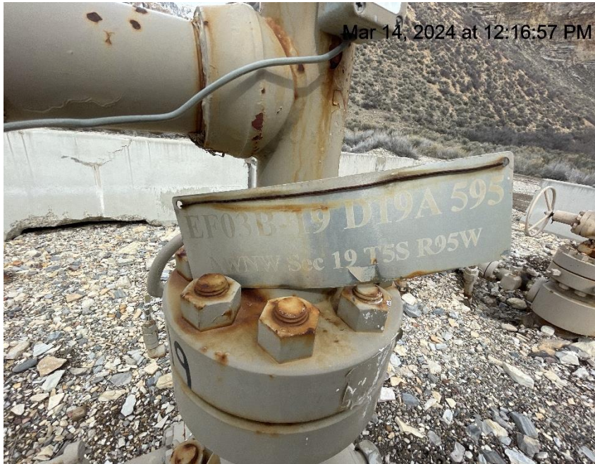
Photo # 88 Wellhead signs lack required info
