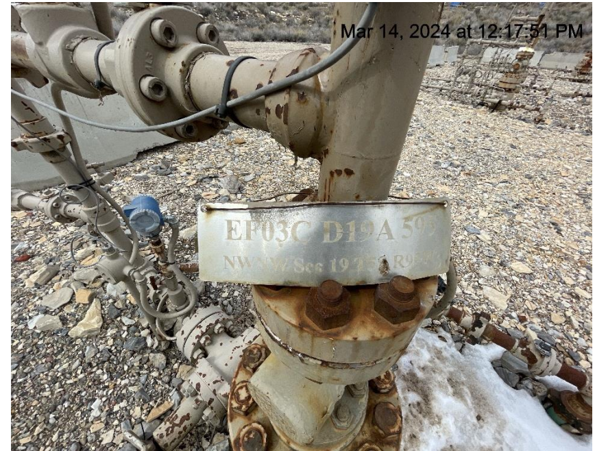
Photo # 87 Wellhead signs lack required info
