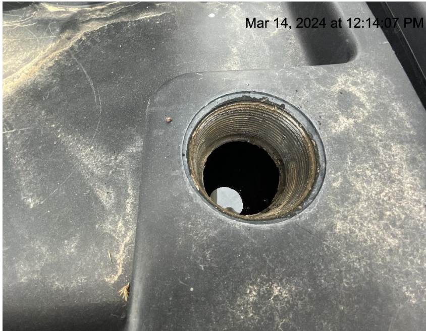
Photo # 90 Chemical containment approximately 3/4 th full of fluid/Failure to maintain chemical BMP/BMP insufficient to contain possible spill
