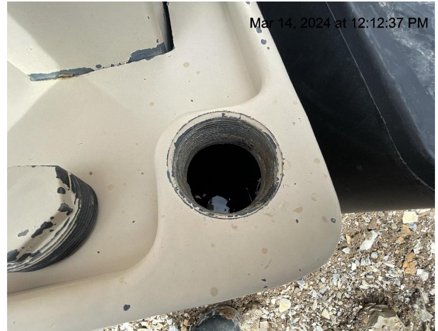
Photo # 91 Chemical containment approximately 5/8 th to 3/4 th full of fluid/Failure to maintain chemical BMP/BMP insufficient to contain possible spill
