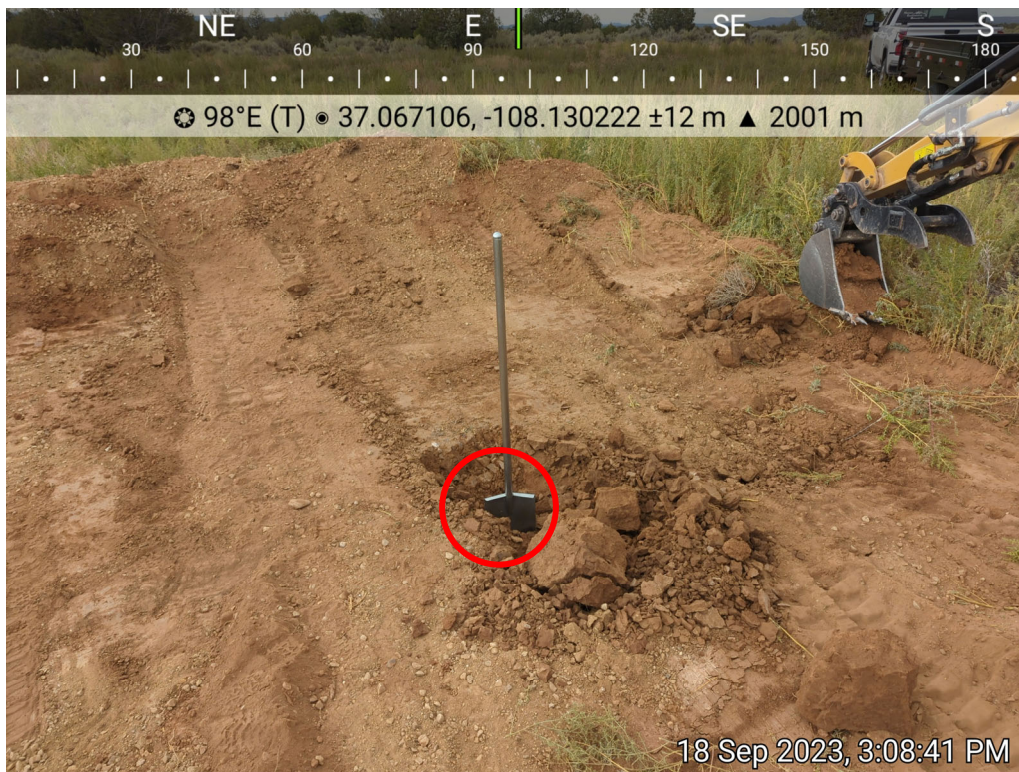
Photo 18: SS15 collected from pothole in the center of AST excavation area, 9/18/2023.
