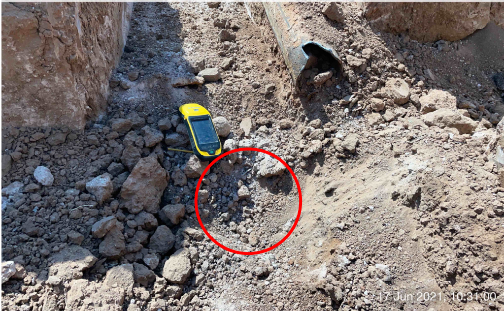
Photo 4: SS04 collected a flowline segment at the Ferguson No. 2 (OWP) F-12, 6/17/2021.
