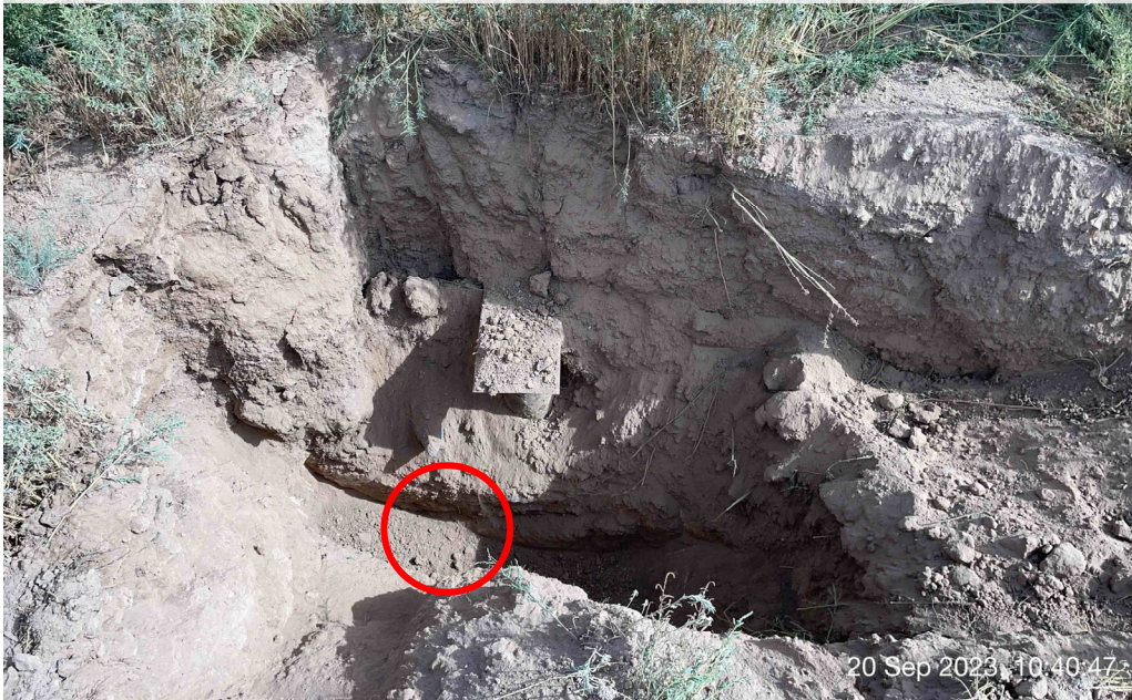
Photo 20: SS09 collected from base of wellhead excavation area, 9/20/2023.
