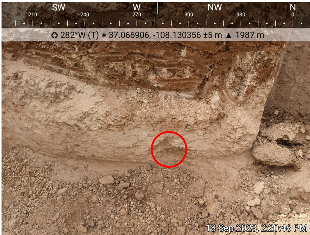
Photo 15: SS13 collected from west sidewall of flowline excavation area, 9/18/2023.
