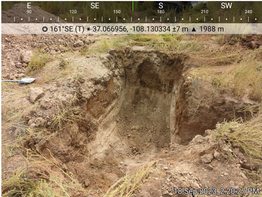
Photo 11: Flowline excavation area, 9/18/2023.
