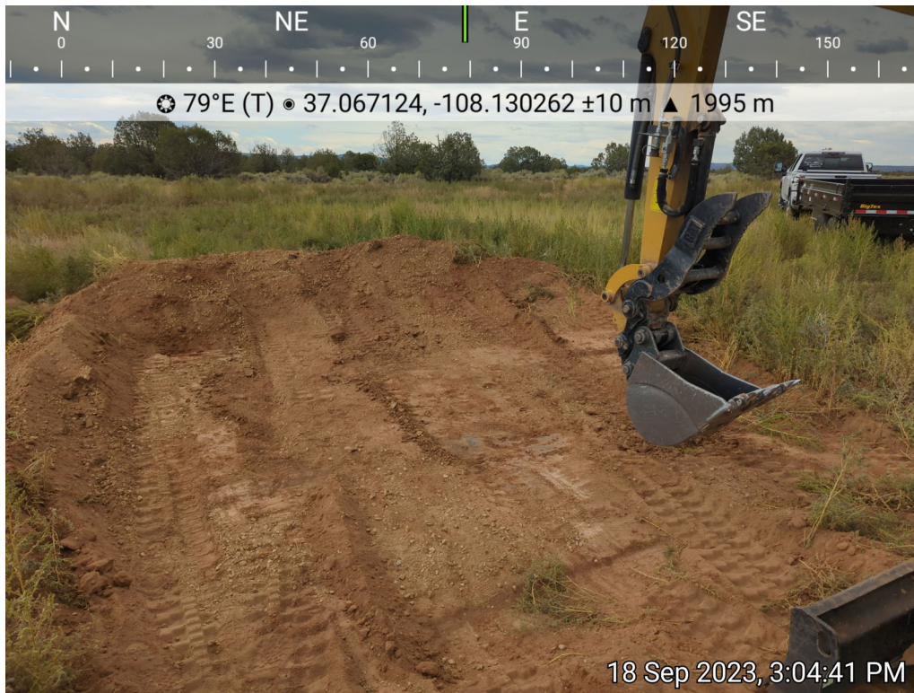
Photo 17: AST excavation area, 9/18/2023.
