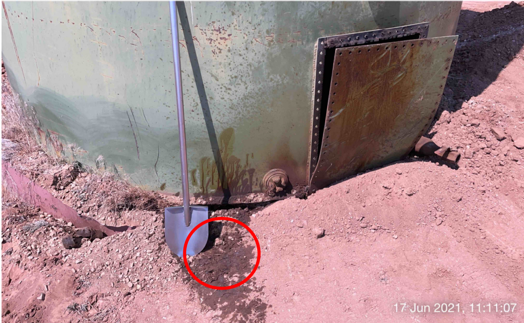
Photo 8: SS08 collected adjacent to AST manway at the Ferguson No. 2 (OWP) F-12, 6/17/2021.
