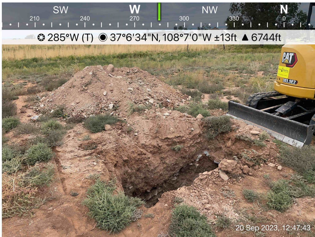
Photo 4: Wellhead excavation area, 9/20/2023.
