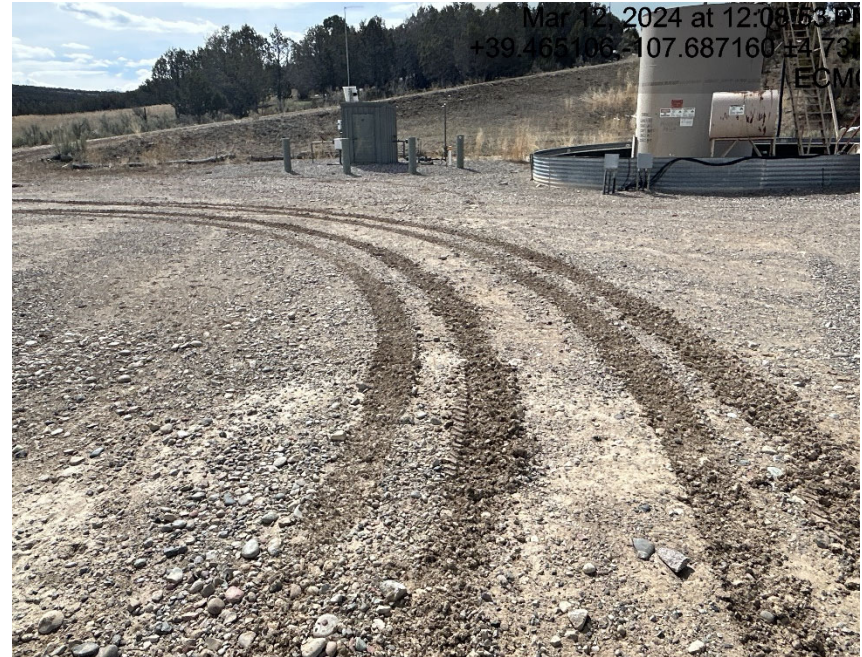
Lack of compaction/ stabilization
