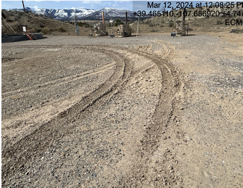
Lack of compaction/ stabilization
