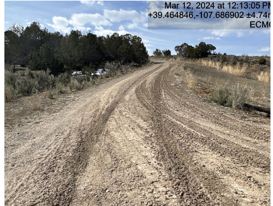
Lacking tracking BMP's
