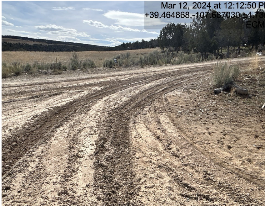
Lacking tracking BMP's
