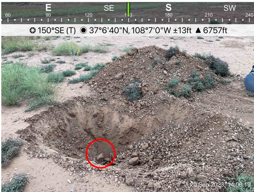
Photo 4: SS03 collected from base of west AST excavation area, 9/20/2023.
