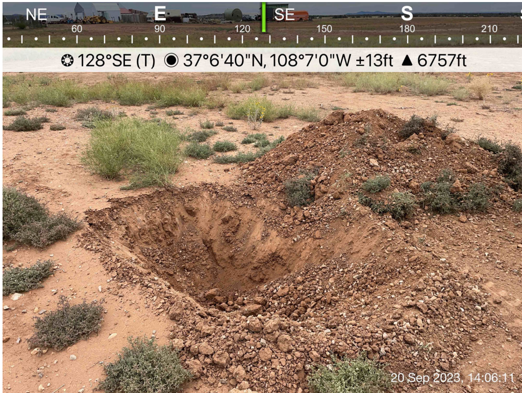
Photo 3: West AST excavation area, 9/20/2023.
