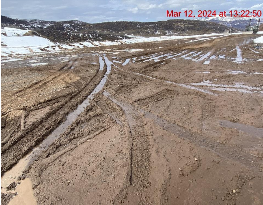
Lack of Stabilization – Photo #09868
