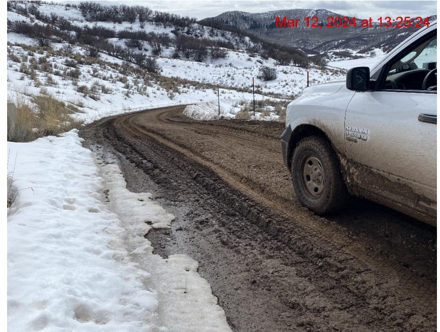
Insufficient Vehicle Tracking BMPs at Location Entrance/Exit – Photo #09873
