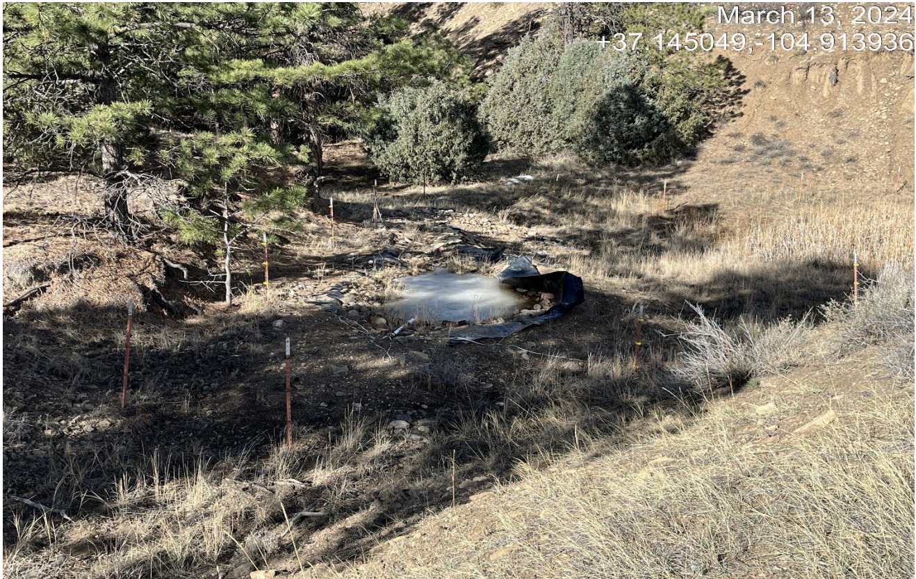
Photo 2. The water discharge point just west of the well is not maintained. The plastic liner is pulled up. The electric fence is in disrepair. T-post and fence should either be removed or maintained.
