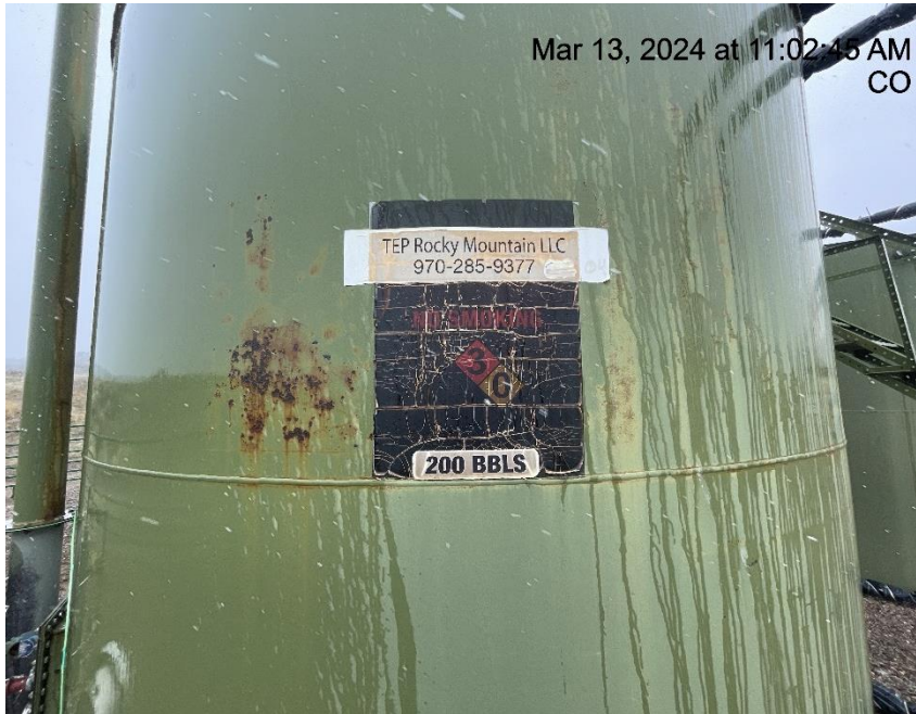
Photo # 9690 Tank label damaged & some required info illegible/does not comply with CECMC tank labeling rules
