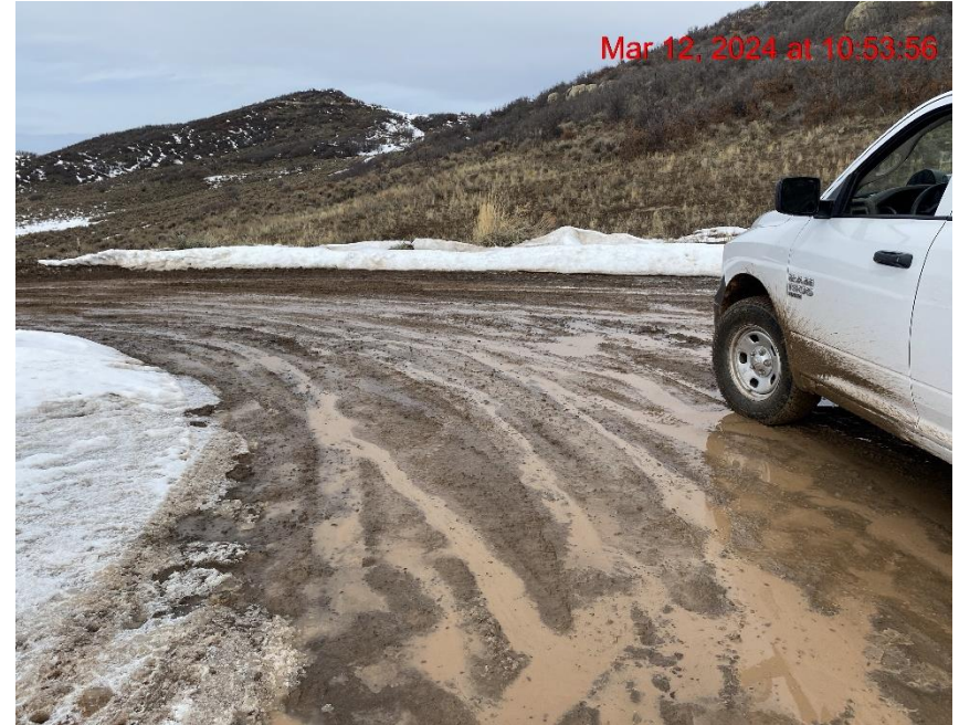
Insufficient Vehicle Tracking BMPs at Location Entrance/Exit – Photo #09796
