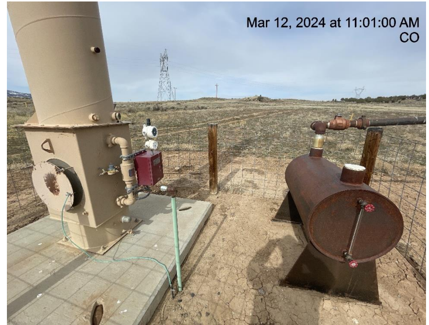
Photo # 9419 Unused equipment/ECD disconnected & not in use
