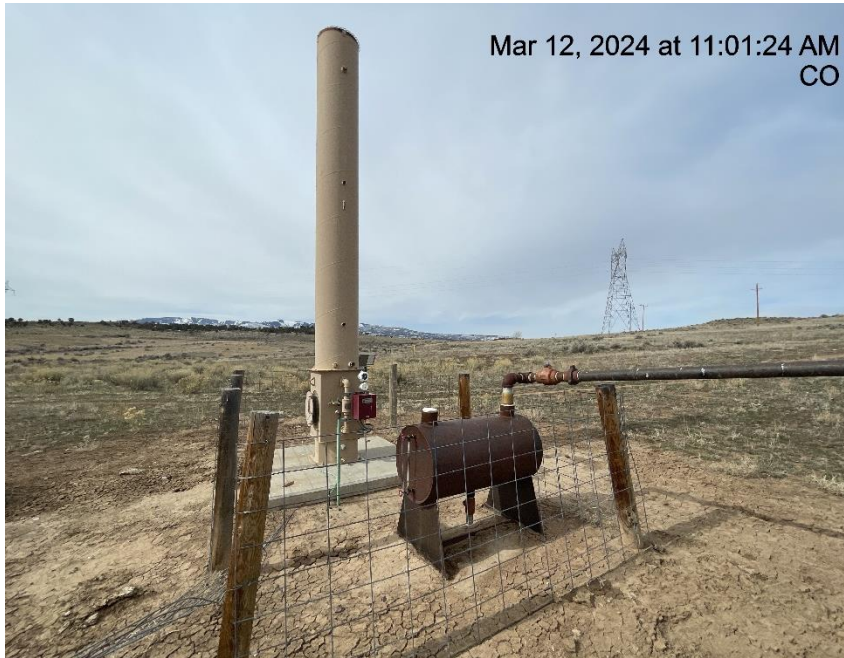
Photo # 9418 Unused equipment/ECD disconnected & not in use
