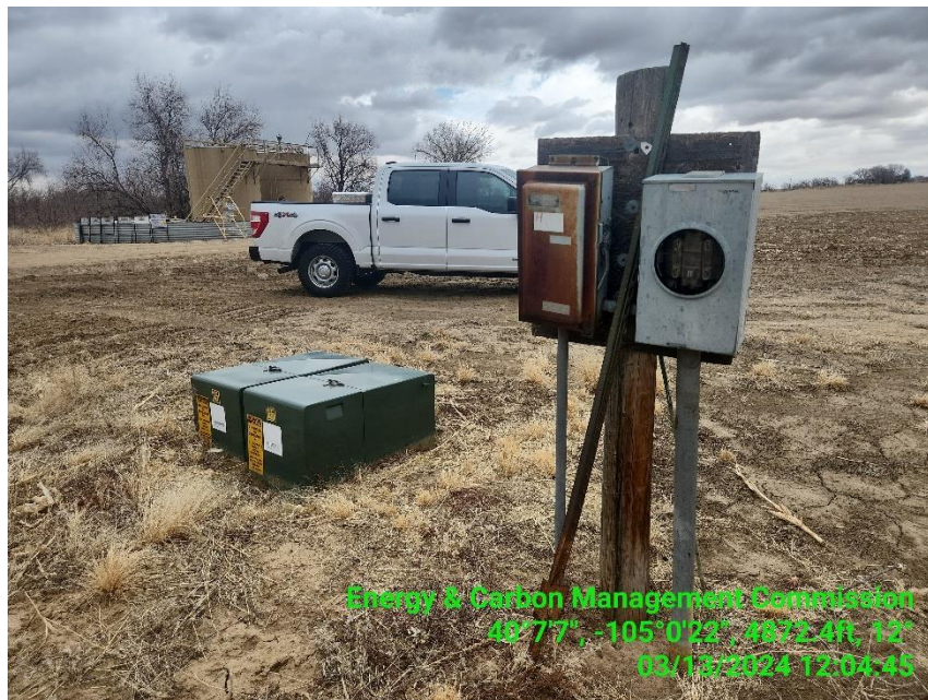
Photo 7 Ancillary equipment is shut off and no meter on the meter box.
