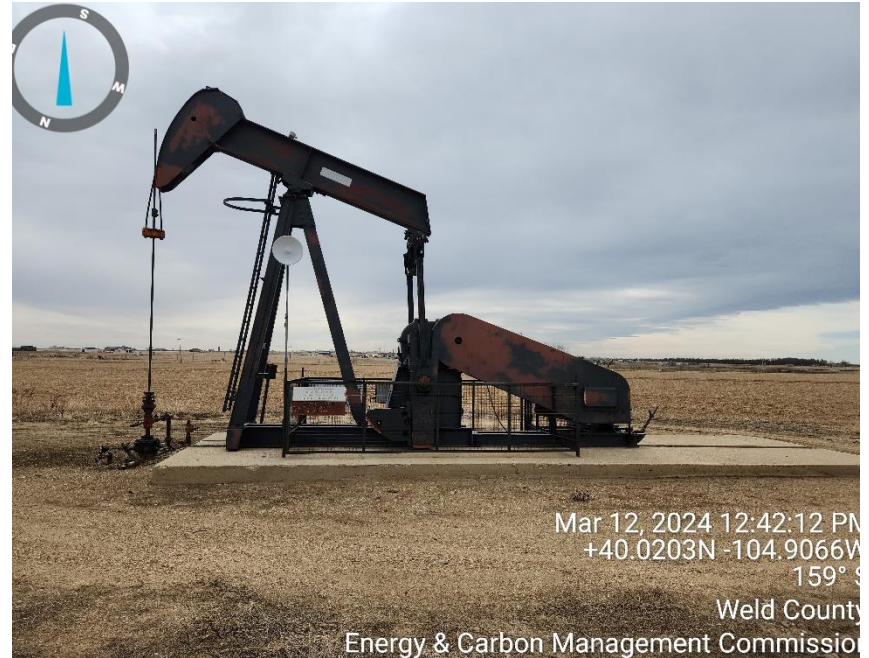
Photo 2 well head and equipment
