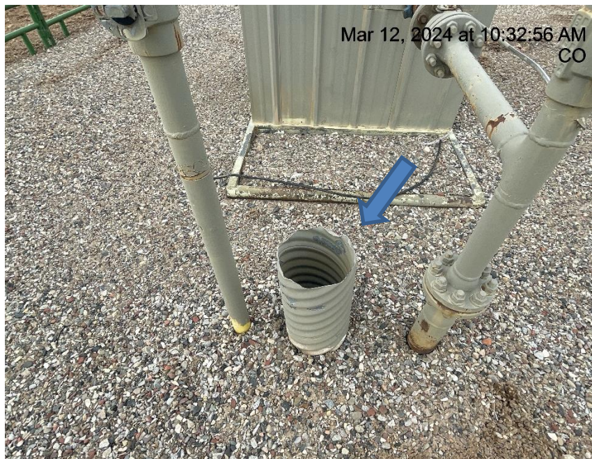
Photo # 9377 Open ended pipe/available for entry by wildlife/wildlife hazard
