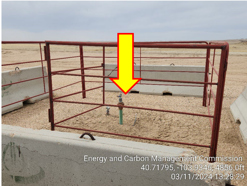
Photo 21 – Unmarked Risers
