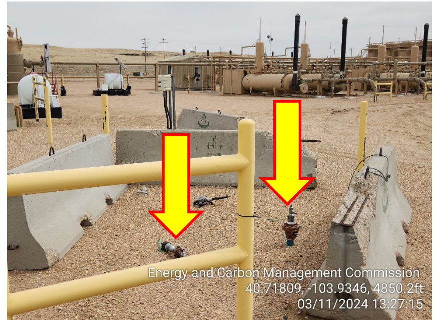
Photo 18 – Unmarked Risers
