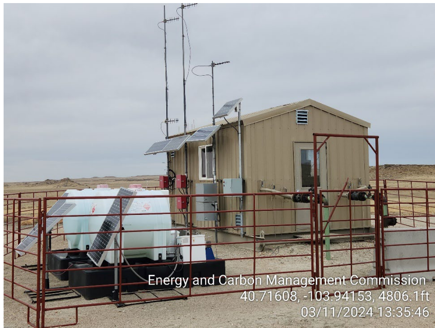
Photo 1 – Gas Lift Injection Meter House
