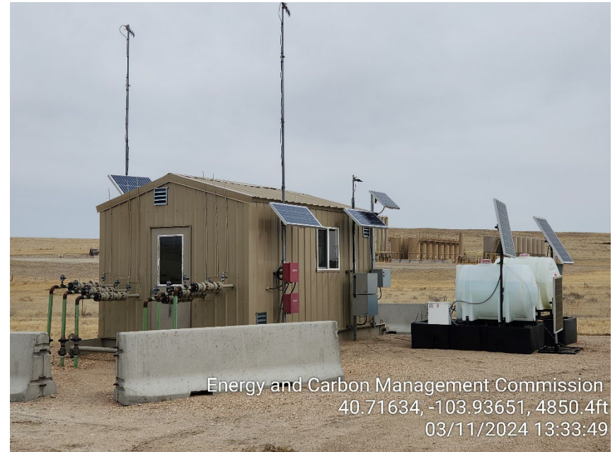
Photo 4 – Gas Lift Injection Meter House
