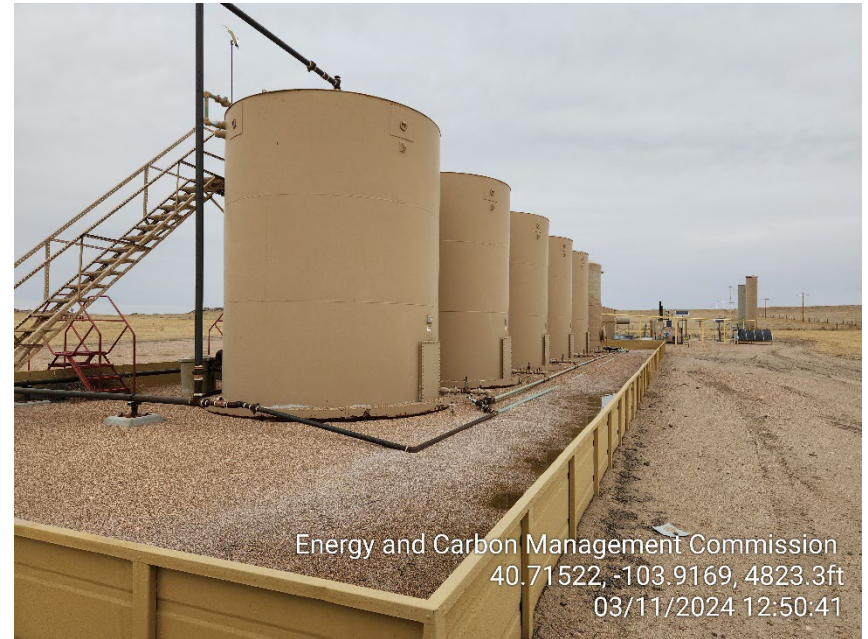
Photo 10 – Tank Battery
