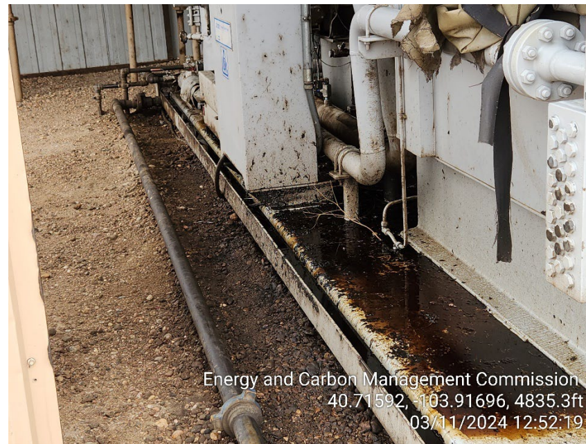
Photo 14 – Compressor – Stained Soil
