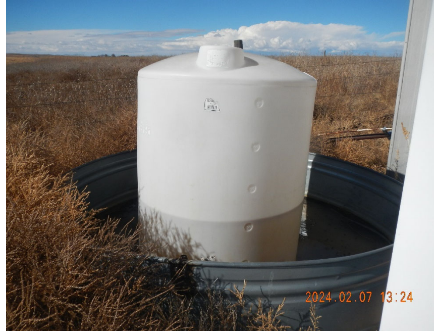
10. Plastic tank in secondary containment.
