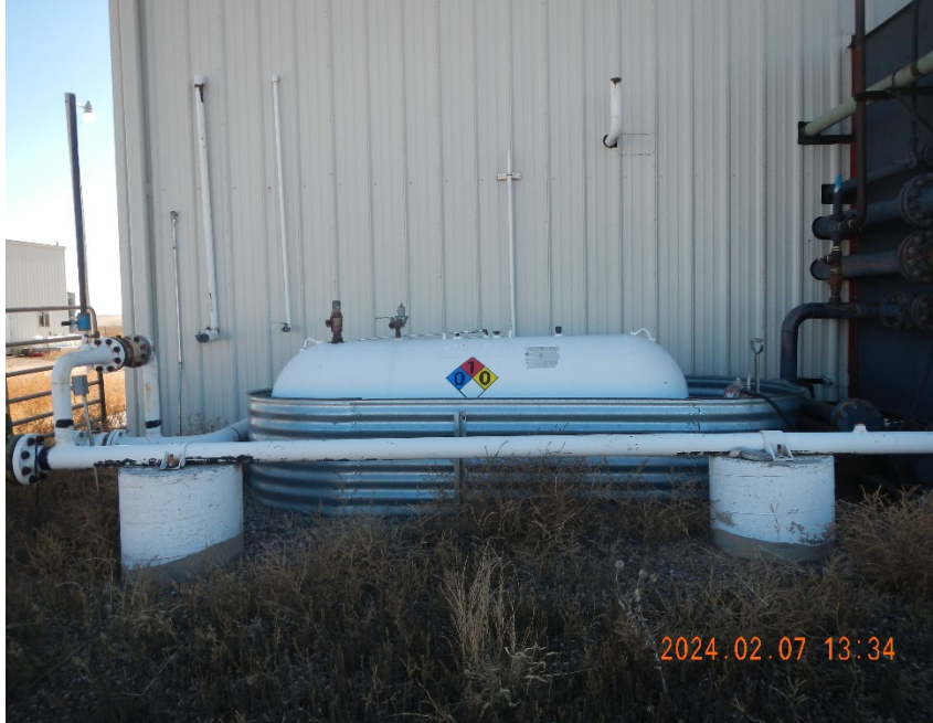
13. Oil tank in secondary containment.
