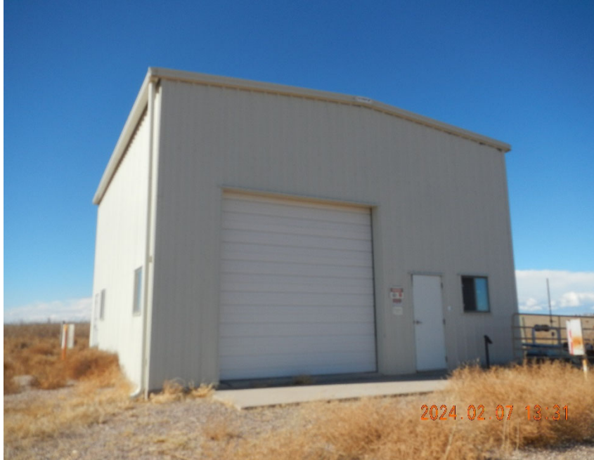
11. Steel built 25' X 30" compressor building.
