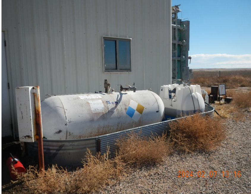
5. Oil tank in secondary containment.
