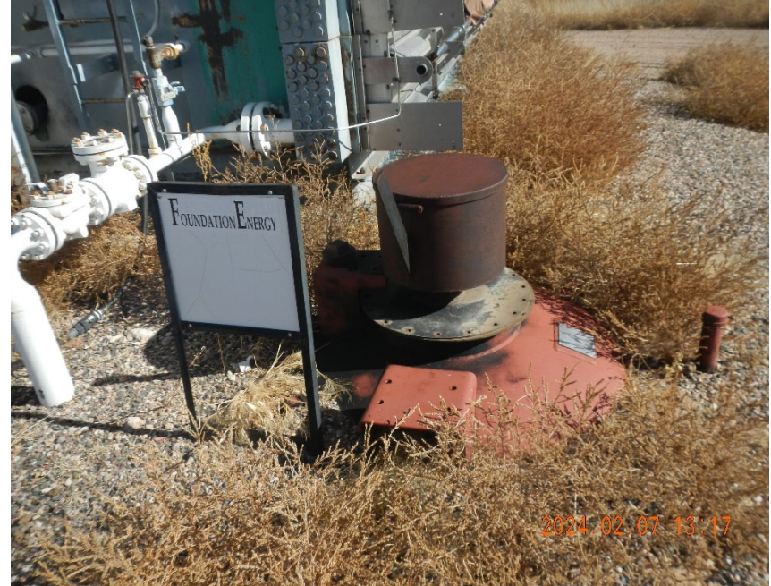
6. Buried steel sump tank outside compressor building.
