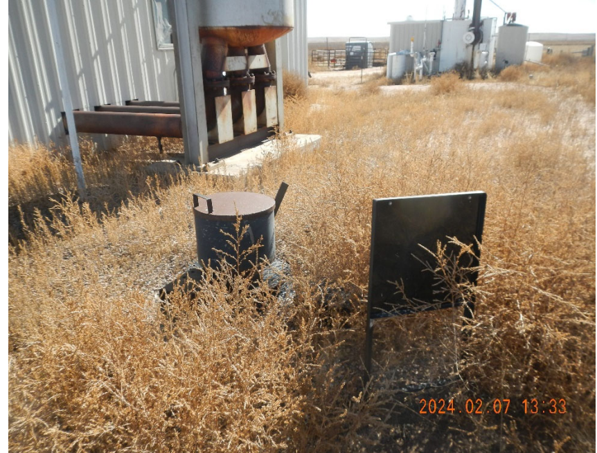
14. Buried sump tank outside compressor building.
