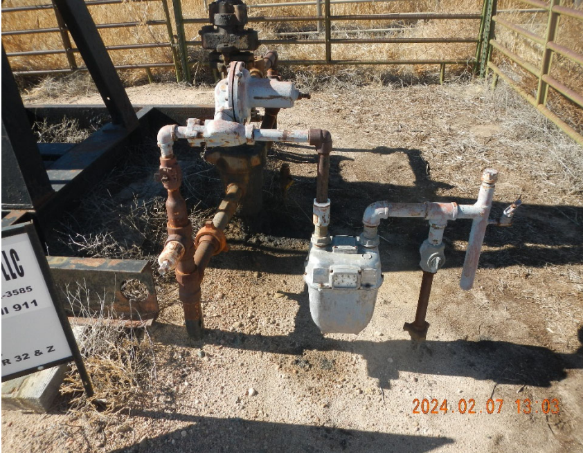
3. View of gas tap off well flowline.
