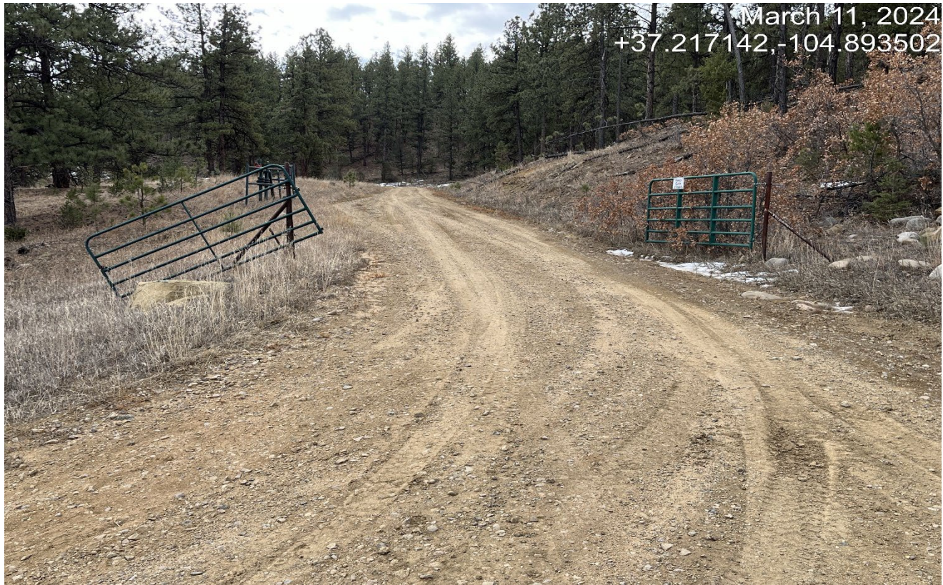
Photo 1. Facing northeast toward the access road. The gate has fallen off the hinges and needs maintenance.
