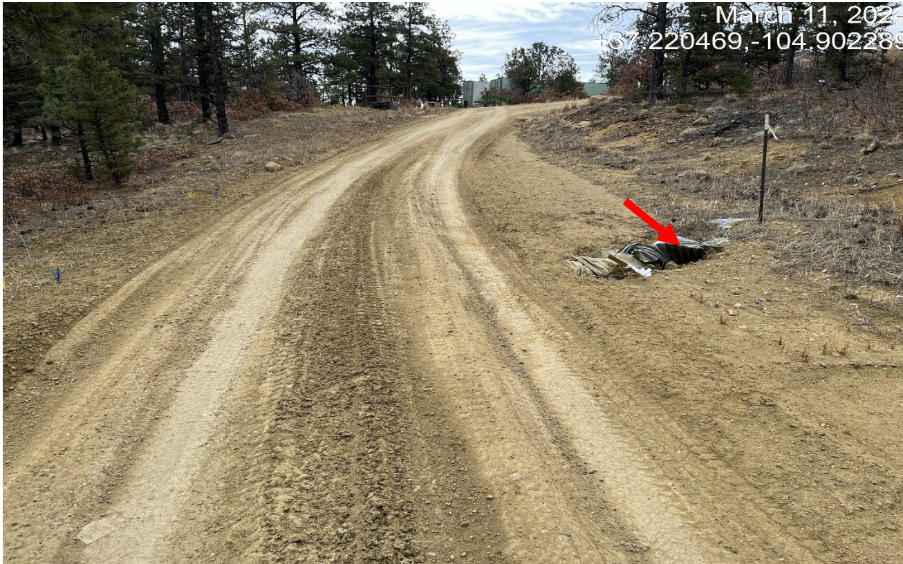
Photo 2. Facing southeast along the access road. This culvert near the wellsite is damaged and needs to be replaced.
