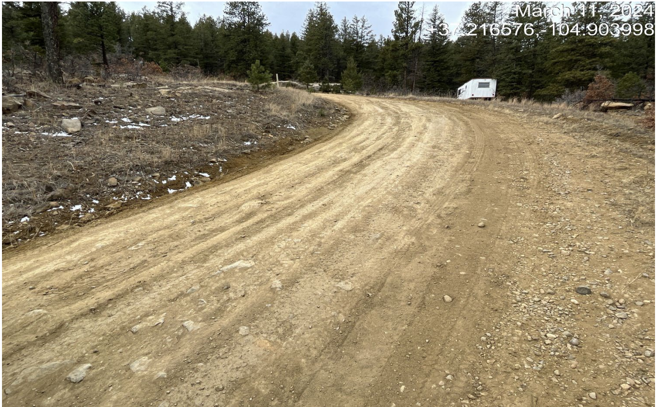
Photo 1. Facing south along the access road. There are signs of vehicle rutting along this switchback area ascending to the location.
