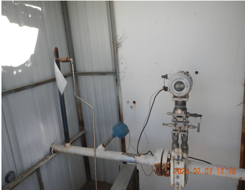
5. Digital gas meter inside meter shed.
