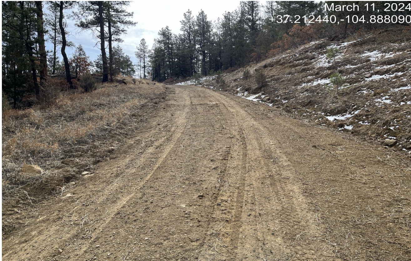
Photo 2. The access road has been bladed and maintained.
