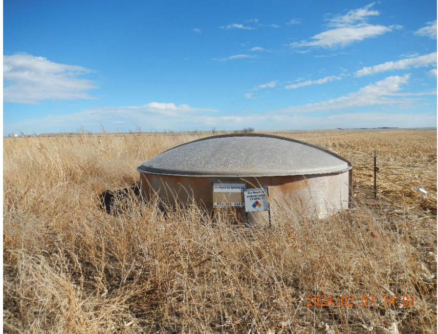
4. Produced water tank.
