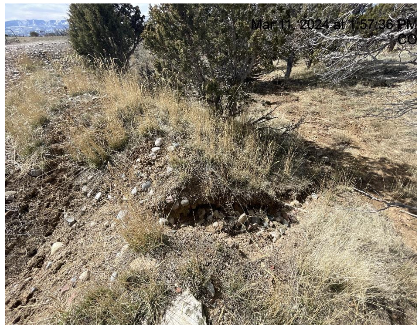
Photo # 9285 Rip Rap run on sediment trap outlet needs maintenance (N/NE area of location)
