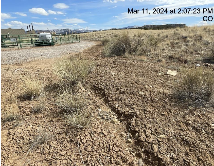
Photo # 9286 Erosion & transport of sediment off location/insufficient BMP's/runoff controls
