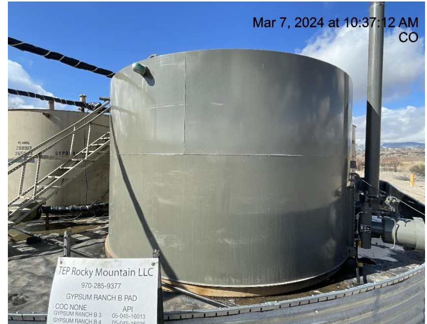
Photo # 9021 Tank lacks required labeling
