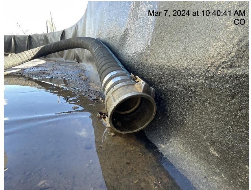
Photo # 9017 Open ended load line
