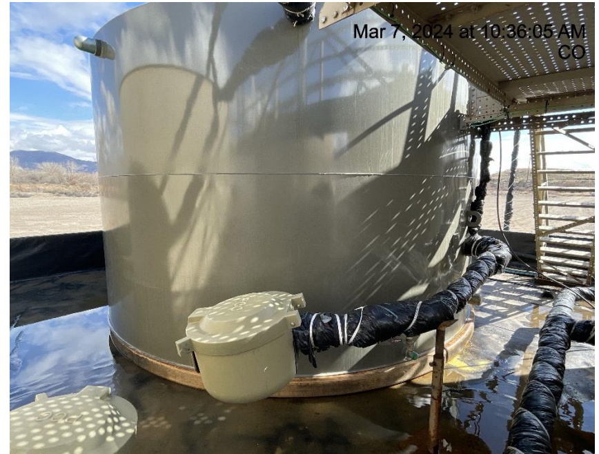
Photo # 9023 Tank lacks required labeling
