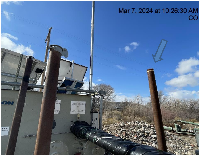
Photo # 9020 Open ended pipe/wildlife hazard
