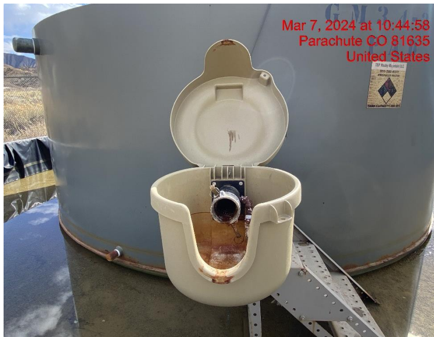
Open-Ended Load Line – Photo #09775
