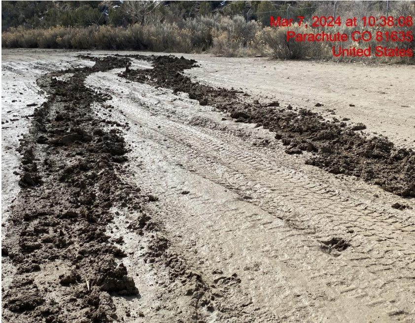
Lack of Stabilization – Photo #09769
