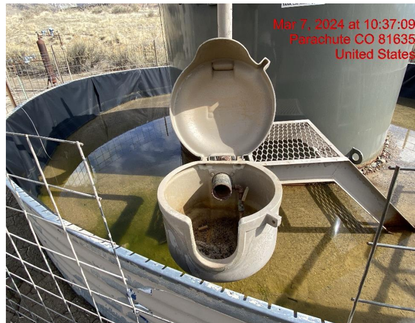
Open-Ended Load Line – Photo #09767
