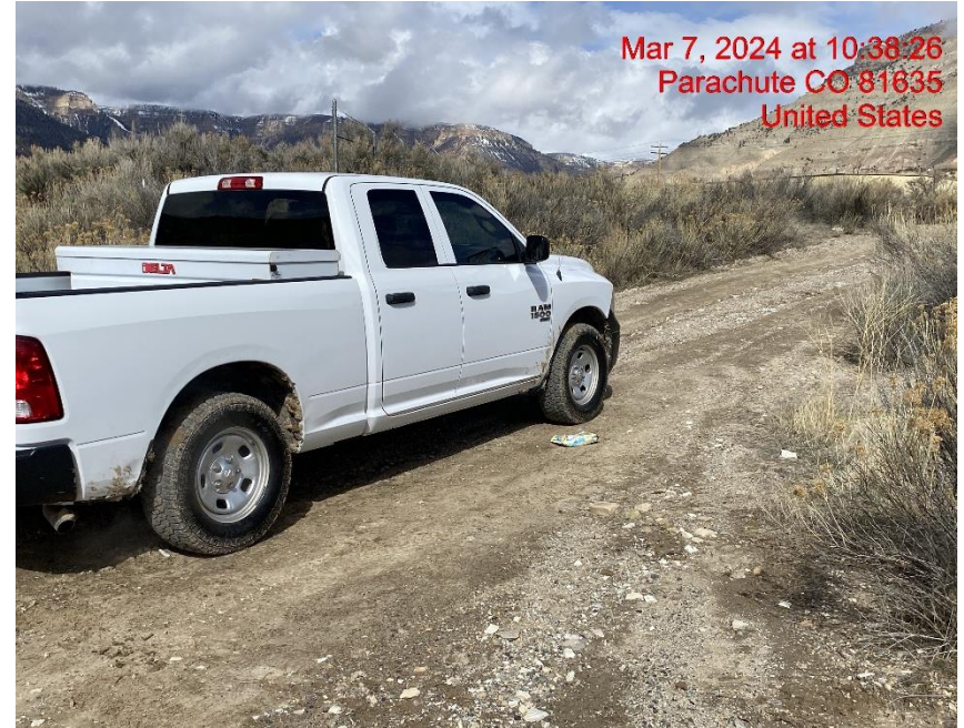
Insufficient Vehicle Tracking BMPs at Location Entrance/Exit – Photo #09770
