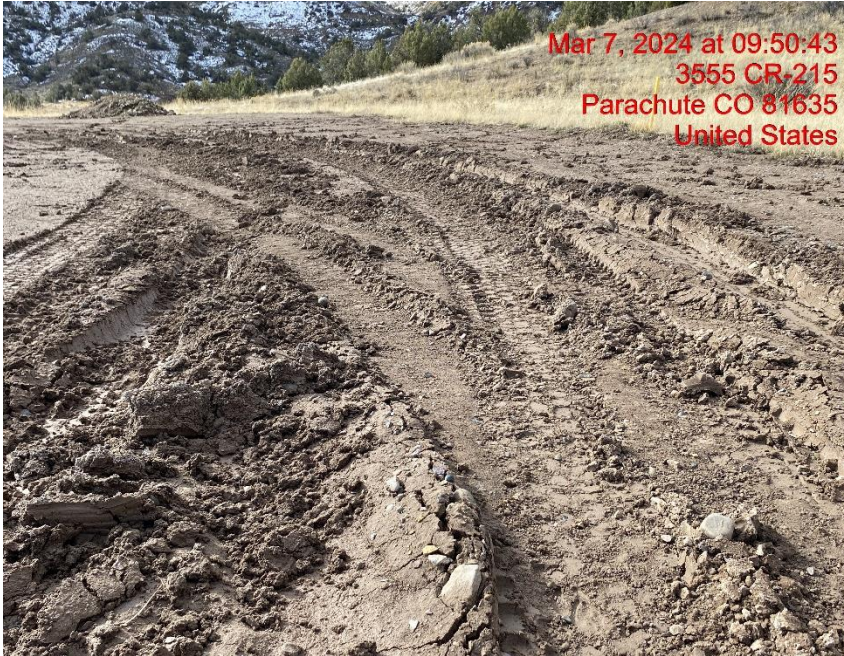
Lack of Stabilization – Photo #09732
