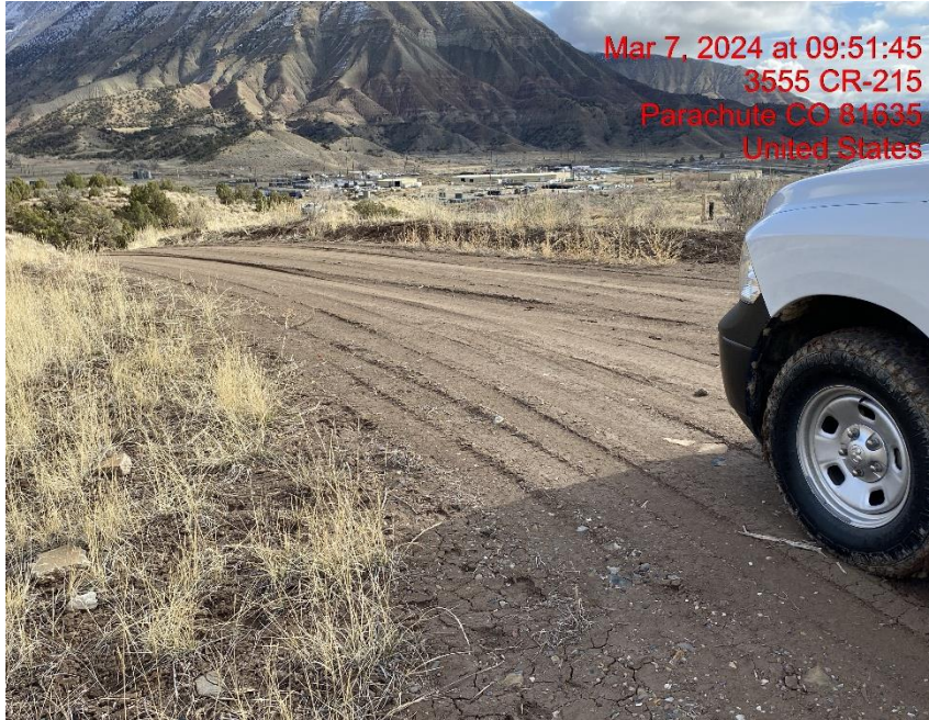
Insufficient Vehicle Tracking BMPs at Location Entrance/Exit – Photo #09734
