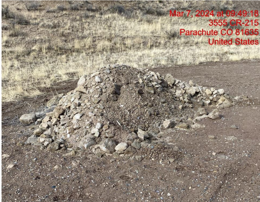
Unprotected Soil Stockpile – Photo #09730
