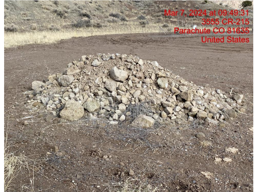
Unprotected Soil Stockpile – Photo #09731
