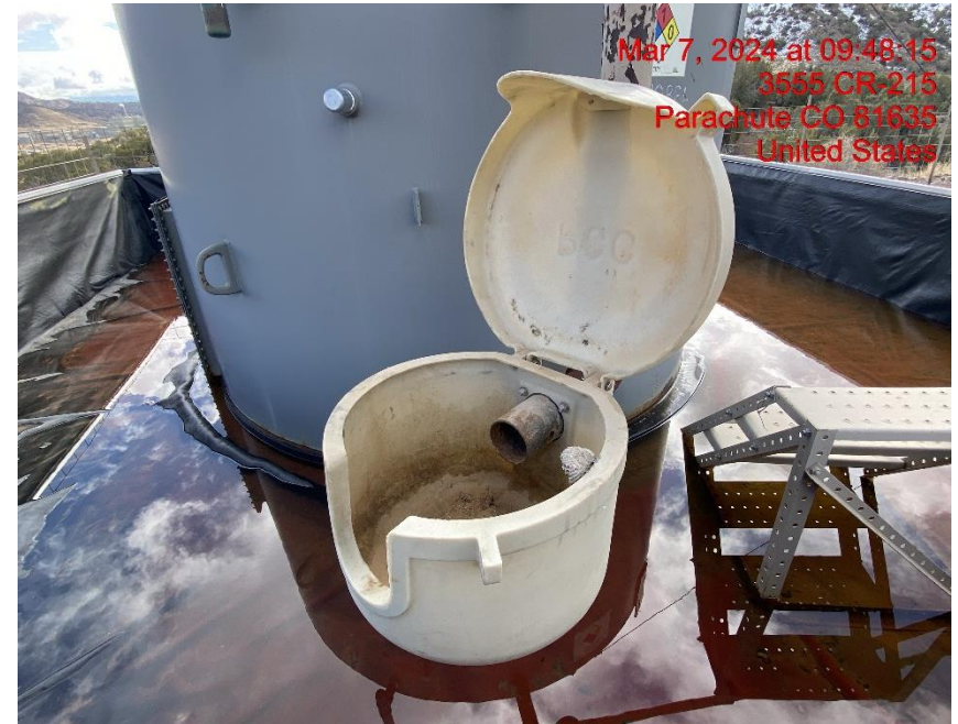
Open-Ended Load Line – Photo #09726
