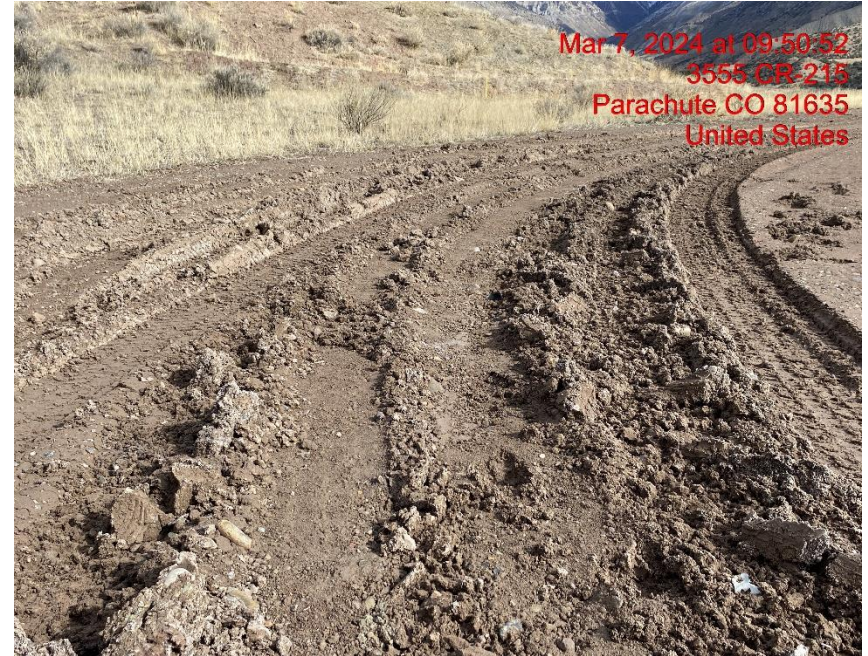
Lack of Stabilization – Photo #09733
