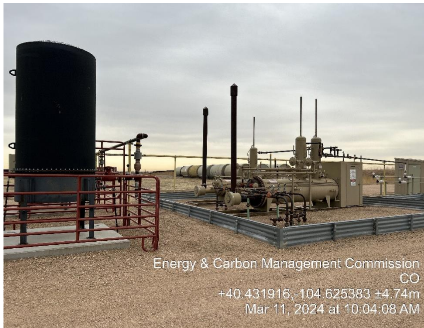
Photo 1 Separator/ECD
