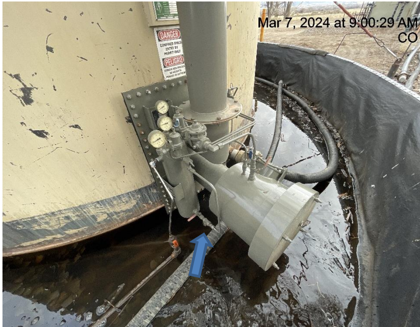
Photo # 8630 PRV vent line terminates in an unsafe manner
