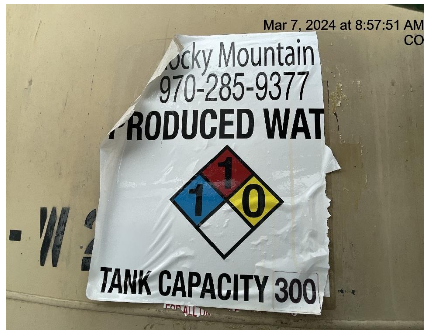
Photo # 8633 Tank label damaged & becoming illegible
