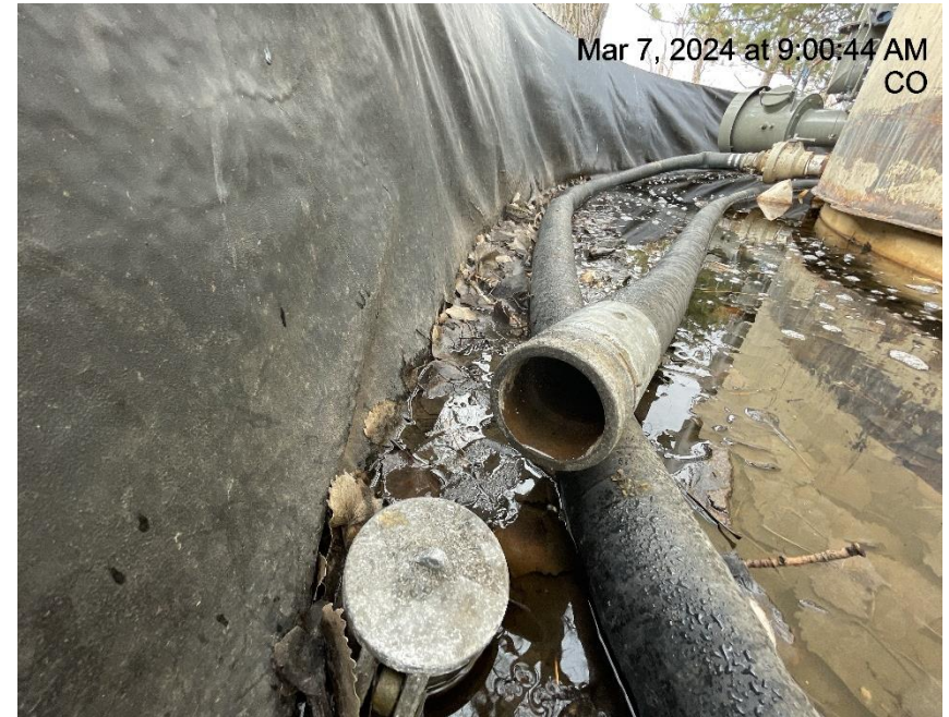
Photo # 8631 Open ended load line
