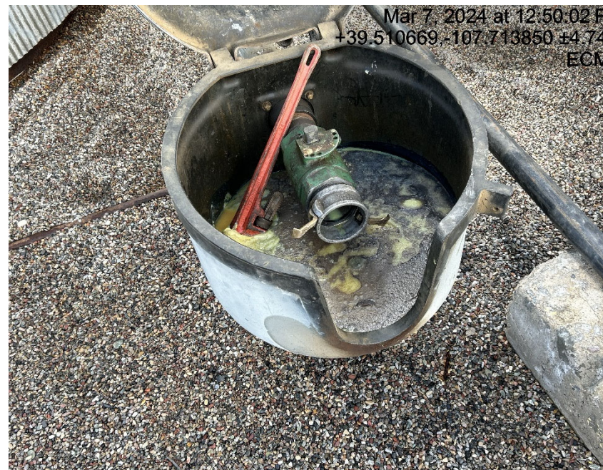
Missing cap/plug and debris
