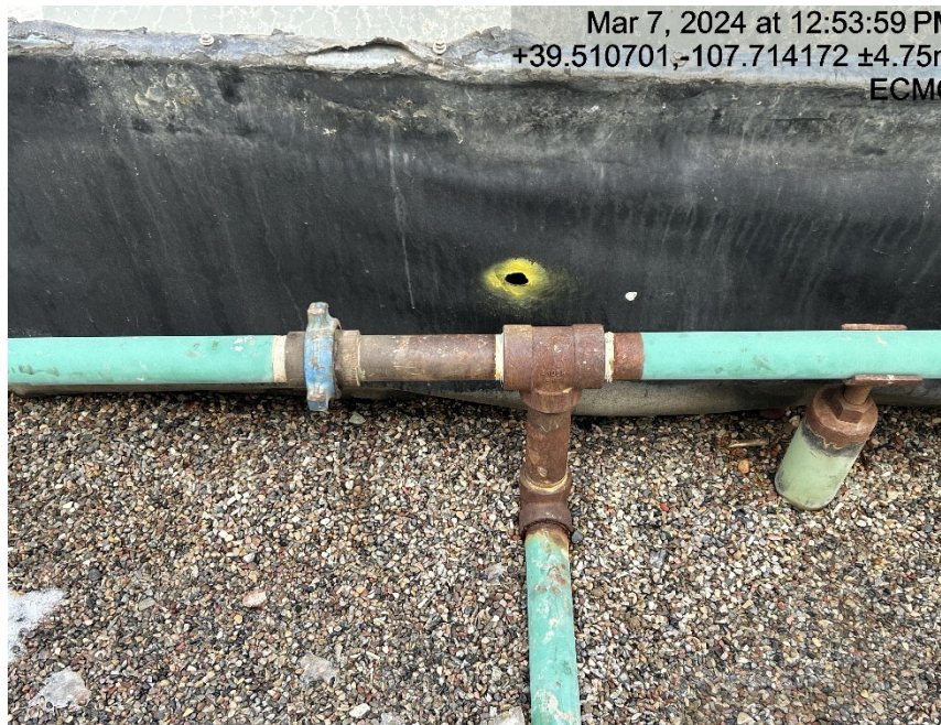
Hole in containment
