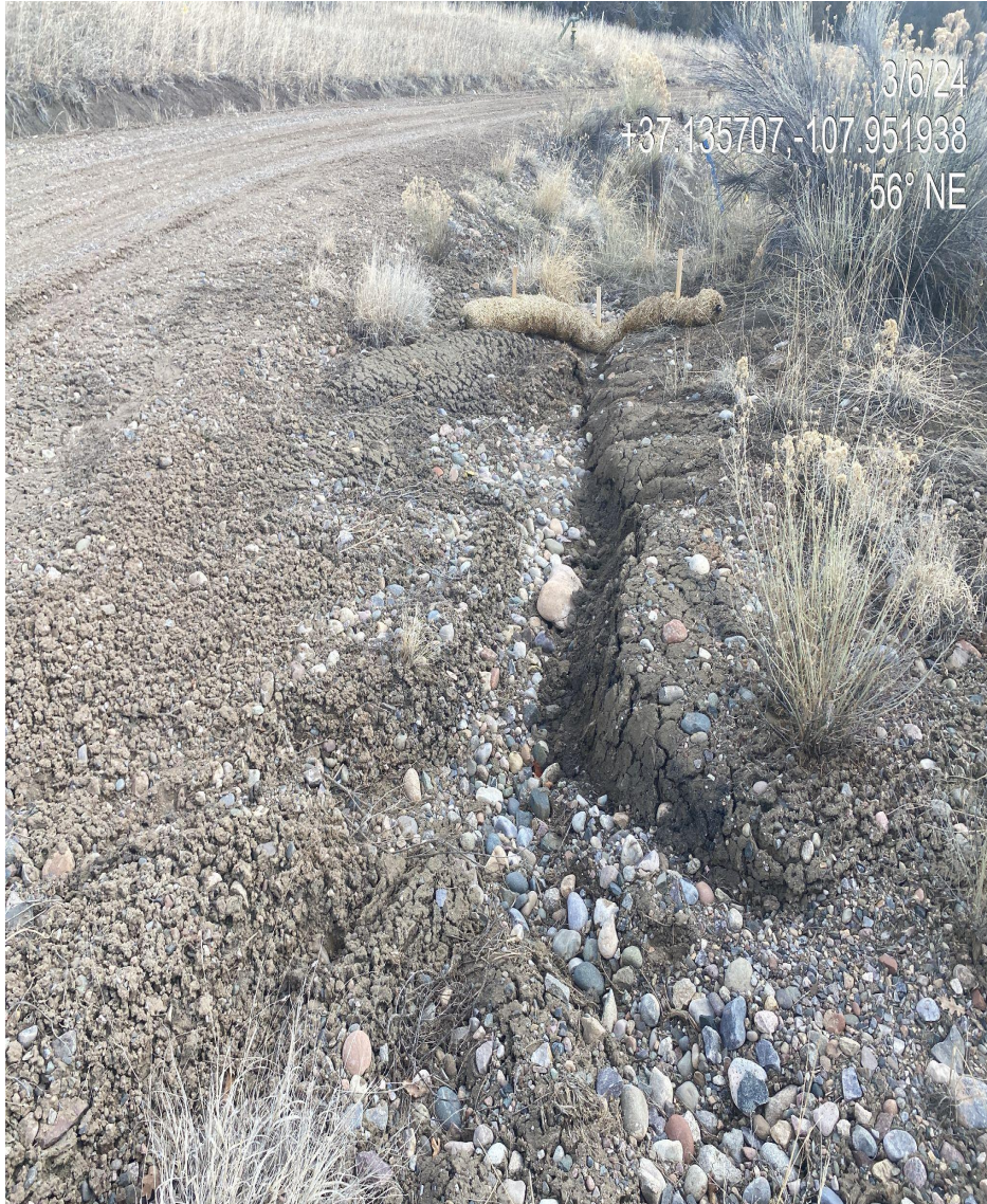
Photo 2. View of gully erosion persisting along the access road and stormwater BMPs that are inadequate.
