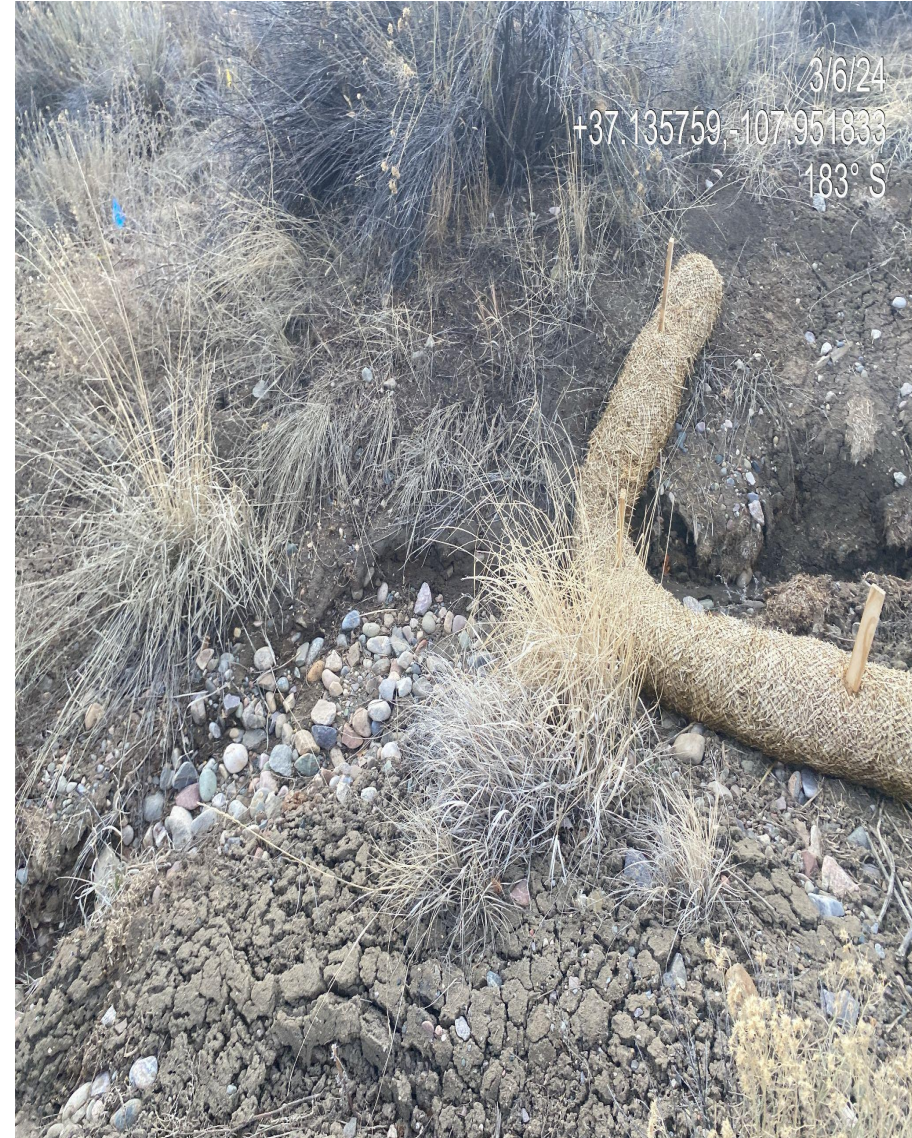
Photo 2. View of gully erosion persisting along the access road and stormwater BMPs that are inadequate.
