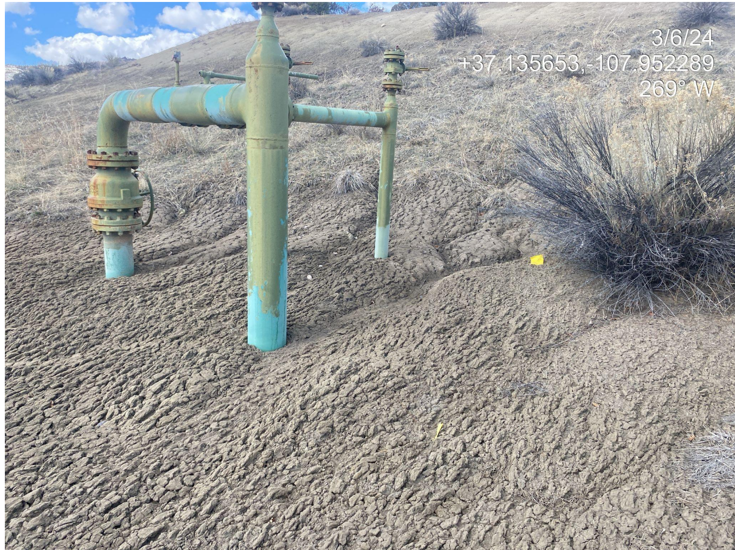
Photo 3. View of additional rill erosion persisting in the western interim reclamation area.
