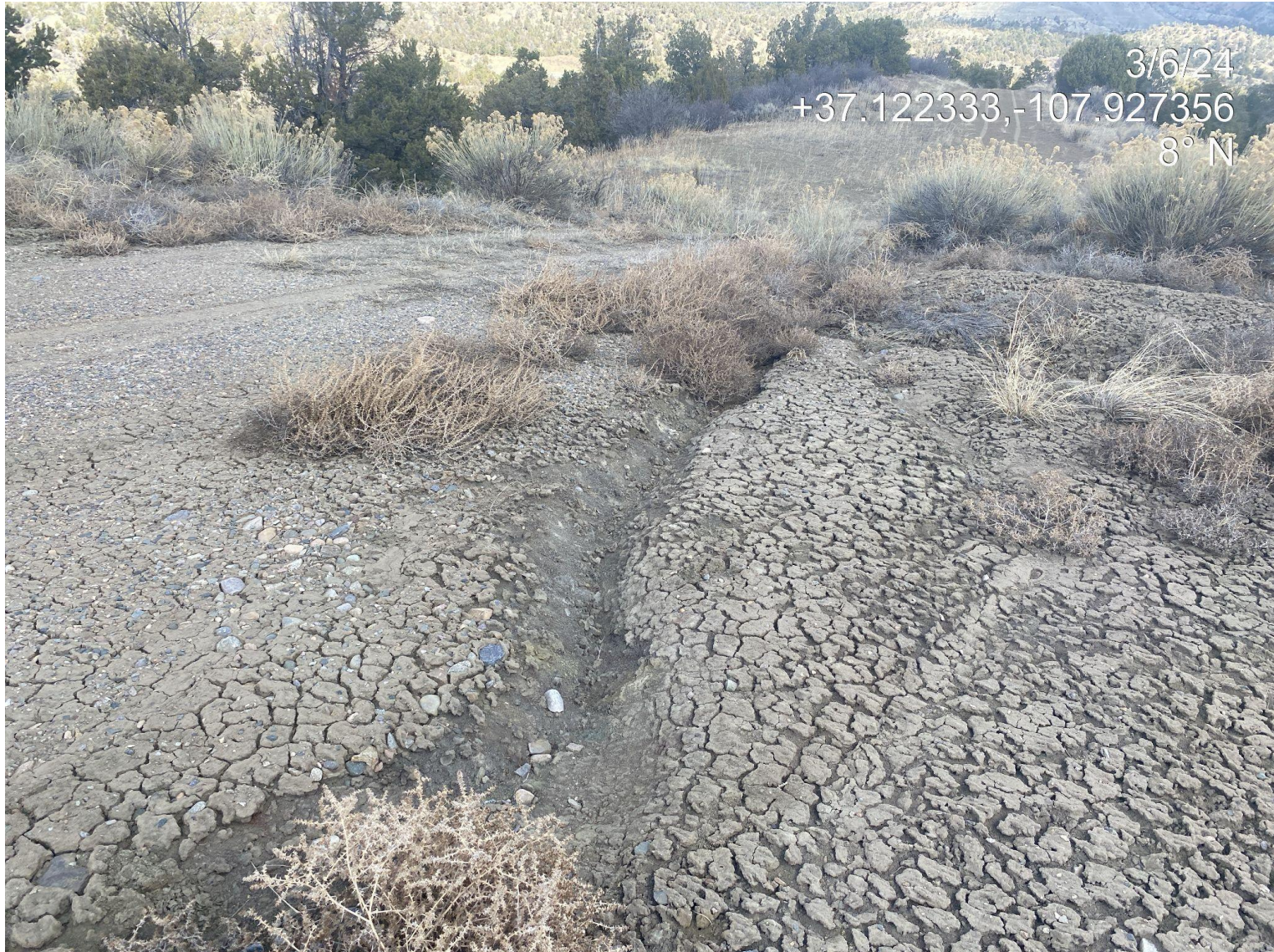
Photo 5. View of additional rill/gully erosion forming at the access point.
