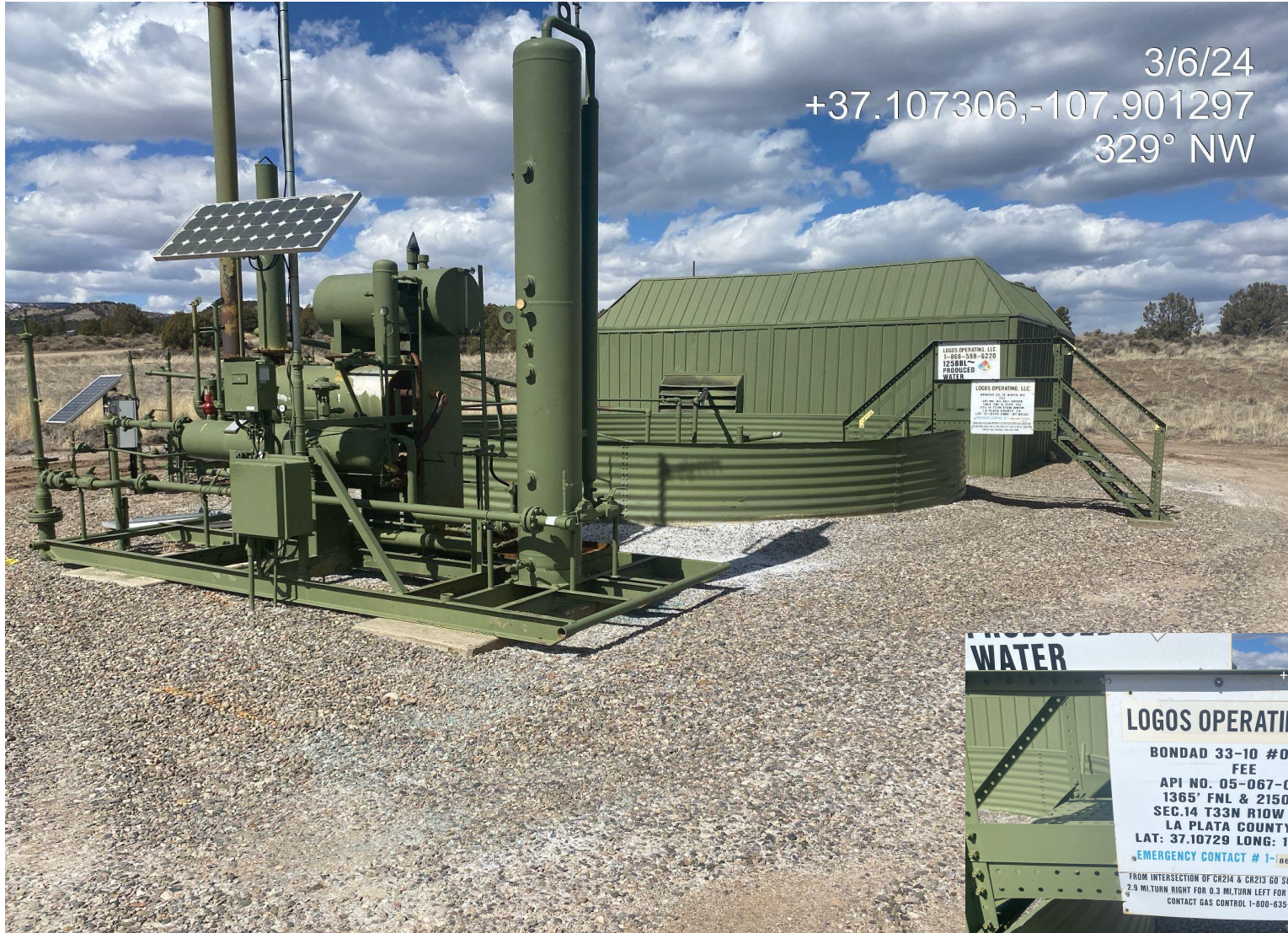
Photo 1. View of the disturbance facing center from the entrance.
