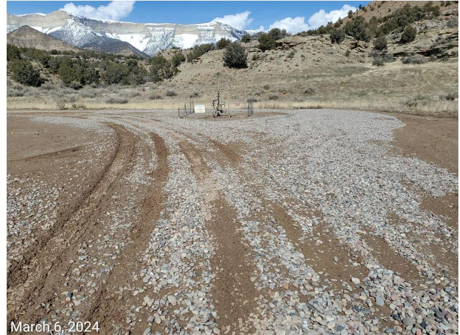
**Photo 1:** Photos 1-2 taken from the working pad surface of the Location. Photos examples showing work to stabilize the working pad surface, as well as to minimize tracking and sediment transport is insufficient. Operator appears to have only placed gravel material over select portions of the Location. BMP alone is inadequate as tracking and degradation issues are recurring; sediment has already filled in large areas of the pad that had been graveled.
