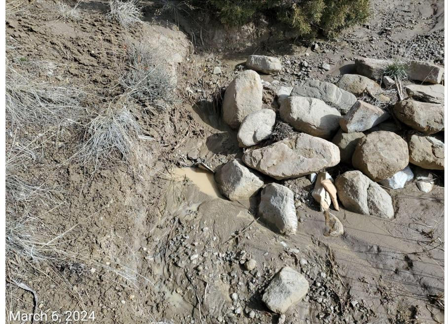
**Photo 2:** Photos taken from the ditch along the north end of the Location. Photo shows stormwater and erosion control BMPs remain missing or insufficient.
