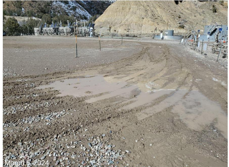
**Photo 1:** Photos taken from the working pad surface of the Location. Photos examples showing work to stabilize the working pad surface, as well as to minimize tracking and sediment transport is insufficient. Operator appears to have only placed gravel material over select portions of the Location. BMP alone is inadequate as tracking issues and degradation issues are recurring; sediment has already filled in large areas of the pad that had been graveled.
