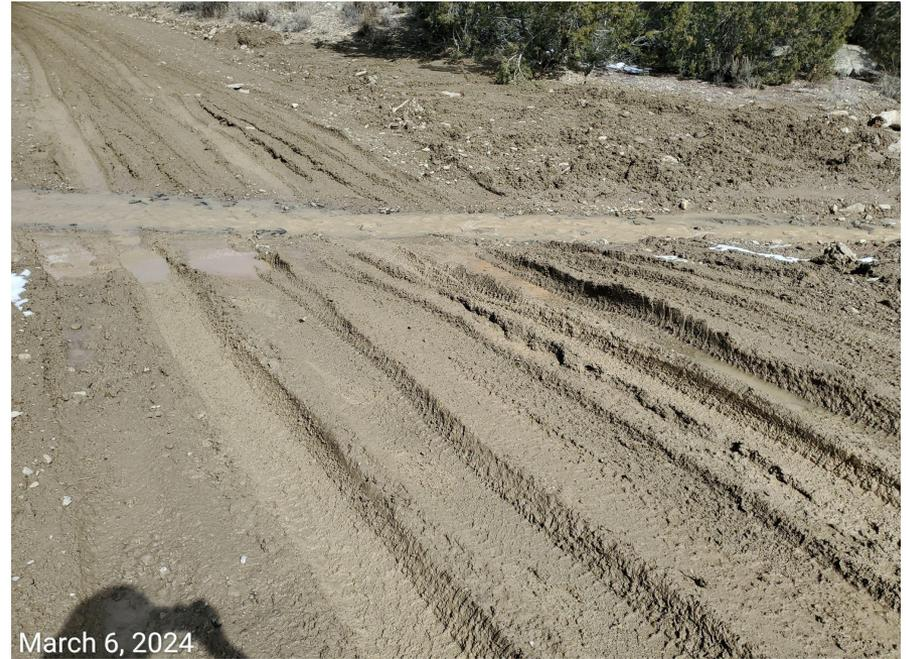
**Photo 3:** Photos 3-4 taken from the access road south of the Location. Photos examples showing that the road has not been constructed with a properly engineered stream crossing; vehicle tracking and degradation apparent at the crossing, impacting a riverine system and Waters of the State. Stream is a direct tributary to the Colorado river.
