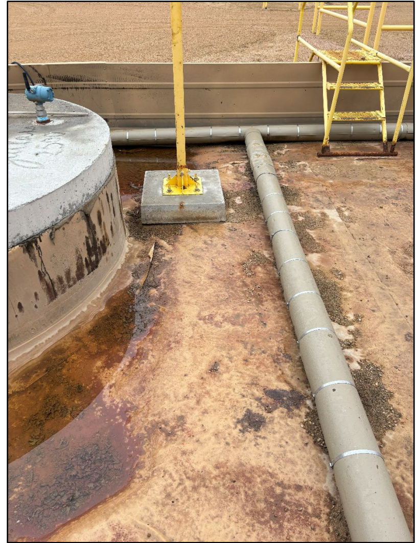
Photo 6: View south of liner containing precipitation around sump
