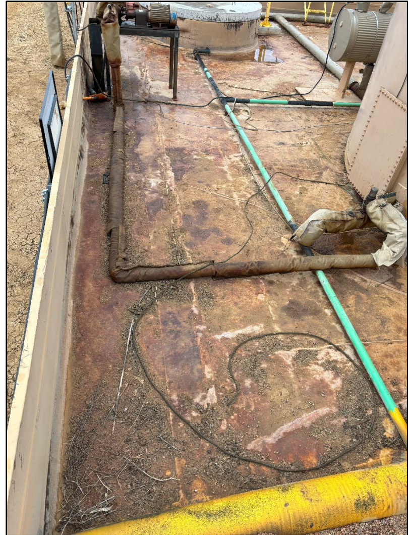
Photo 2: View south of liner, sump, AST, and recirculating pump
