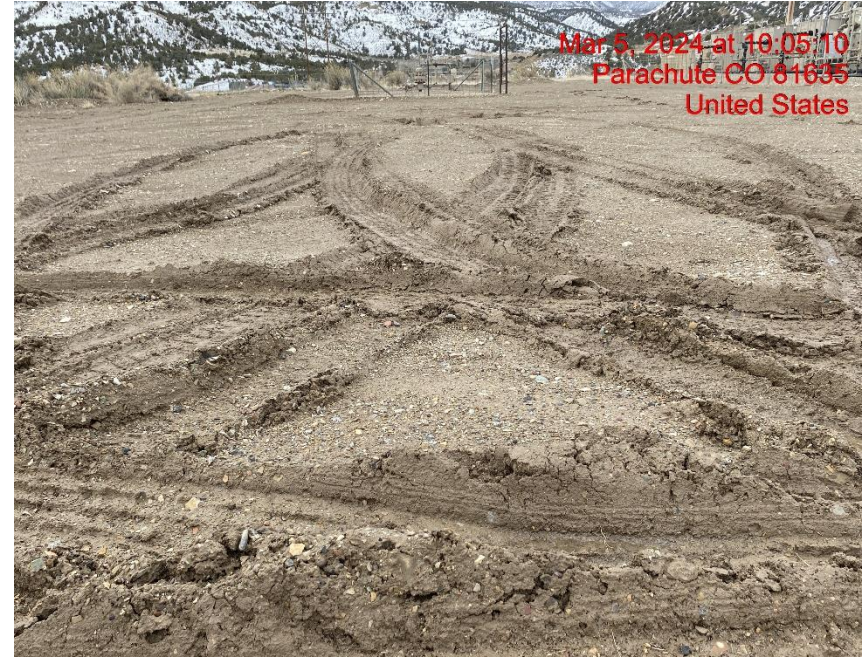
Lack of Stabilization – Photo #09696
