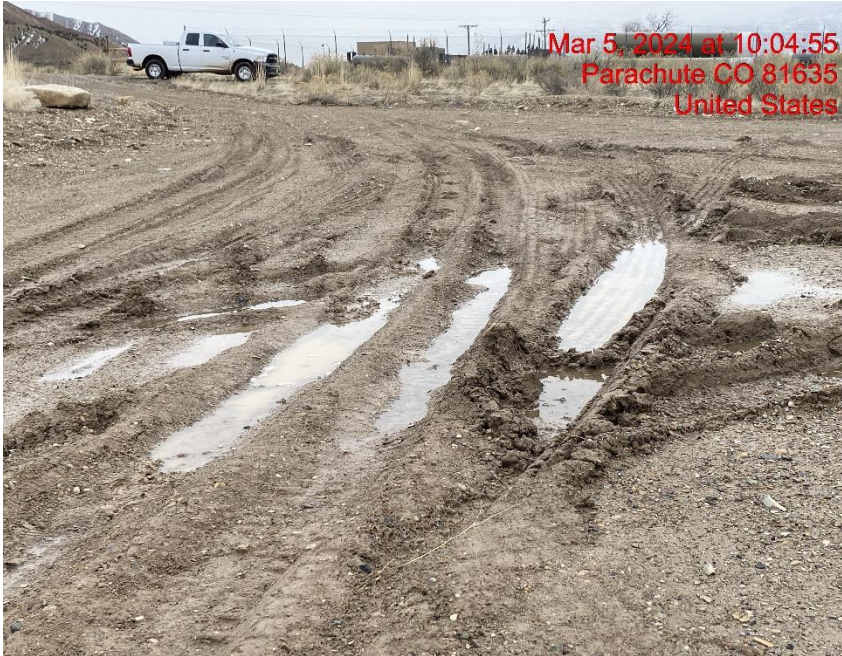
Lack of Stabilization/Insufficient Vehicle Tracking BMPs at Location Entrance/Exit – Photo #09695
