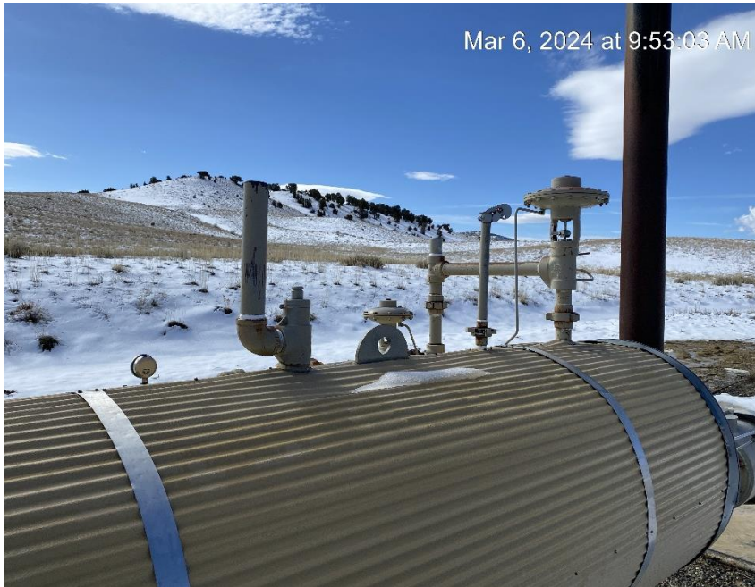
Relief riser missing rain cap
