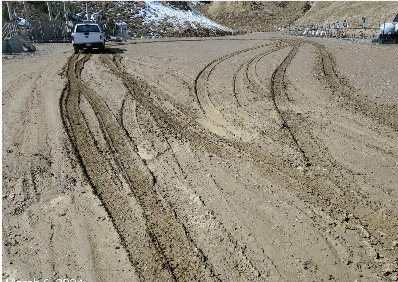
Photo 2: BMPs to stabilize the working pad, as well as to minimize erosion, degradation and sediment transport (tracking) remain missing or insufficient.
