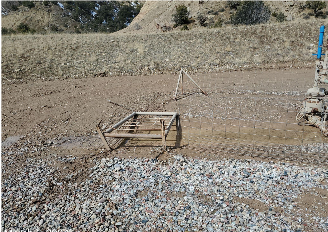
Photo 3: Photo example showing fence at wells is in disrepair.
